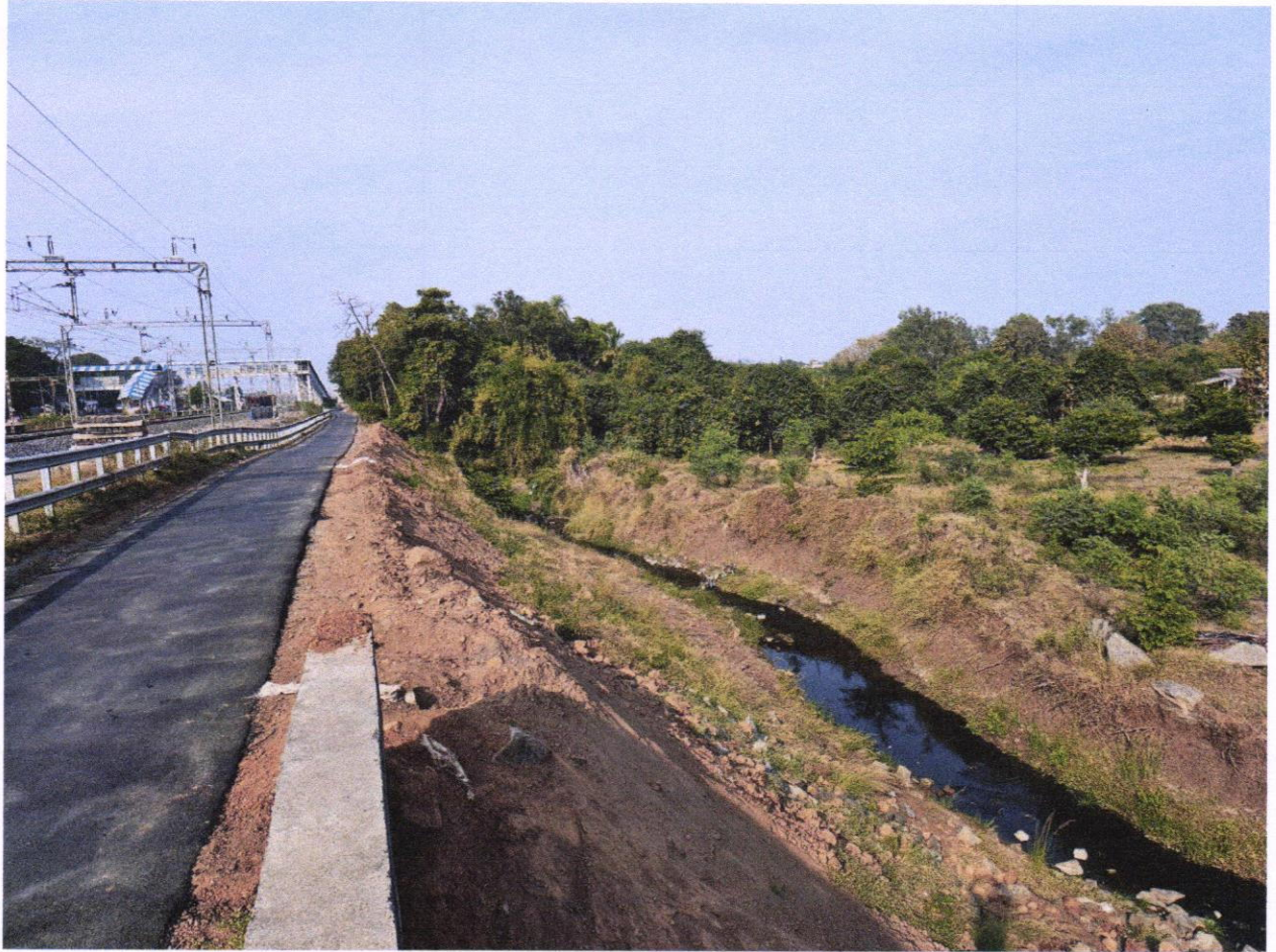
4. Balakhadi Drain which has to be made of Concrete by DFCCIL
